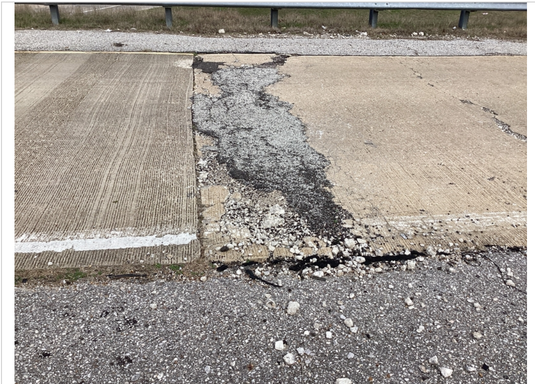
Approach #2 pavement failing patch
