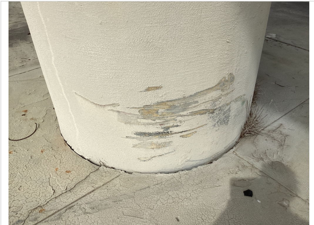
Abrasion on column. Bent 1
