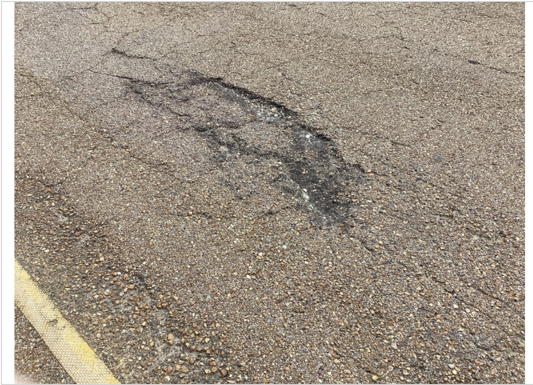
Top deck span #3 spalling
